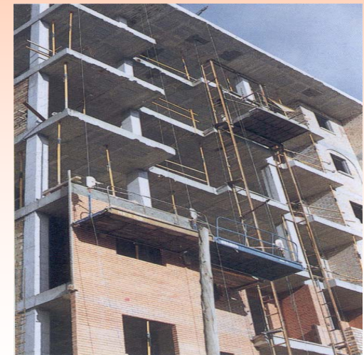
Slab construction with Ceiling Blocks
