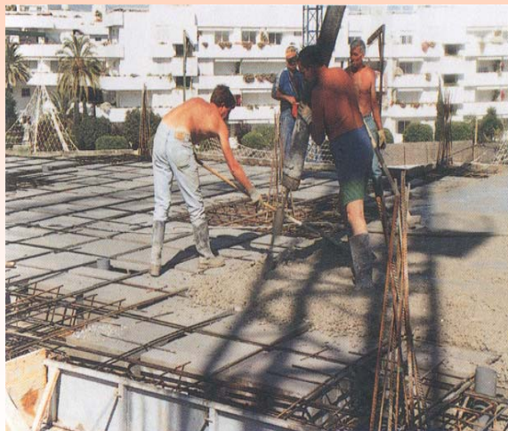
Slab construction with Ceiling Blocks
