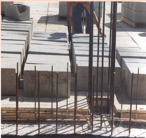
Slab construction with Ceiling Blocks
